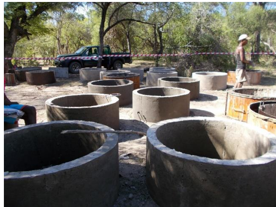
Water well construction underway
